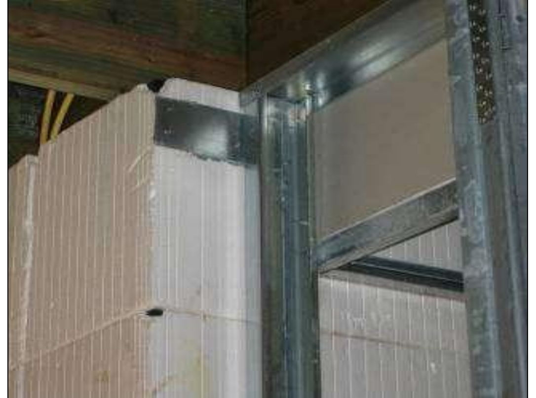
Light-gauge Metal Framing
